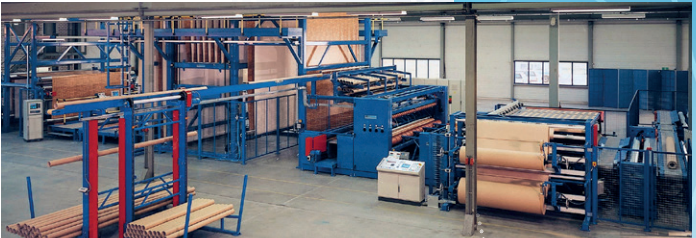
End of a vinyl production line M 6300
