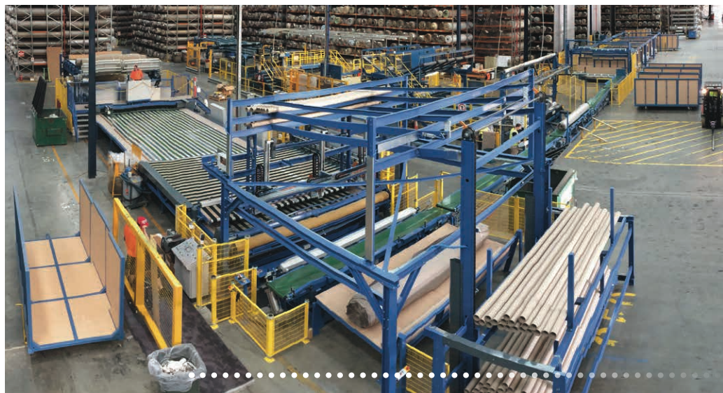
Overview of new cut-length line, conveyor system and sorting system
